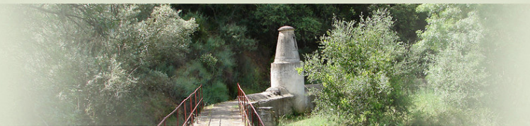
Section of the Aquaduct between S. Bento de Castris and Metrogos, 7 Km long. Totally rebuilt in 1892 after the collapse of the old XVI th aquaduct. The present section is the basis of the aquaduct track.
