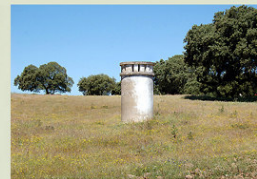
Section of the Aquaduct between Graça do Divor and the Metrogos, 7 Km long.
